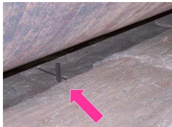
Figure 4 – Location of furnace control thermocouple adjacent to a cast pipe in an annealing furnace
