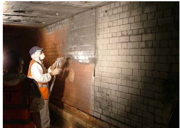
Figure 5 - EMISSHIELD® being sprayed in a tunnel kiln
